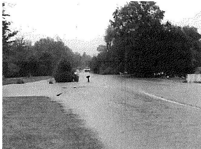
Inundation Flooding on Brooklyn Road - 2011
