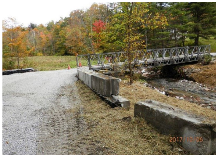
Parker Road Temporary Bridge - 2017
